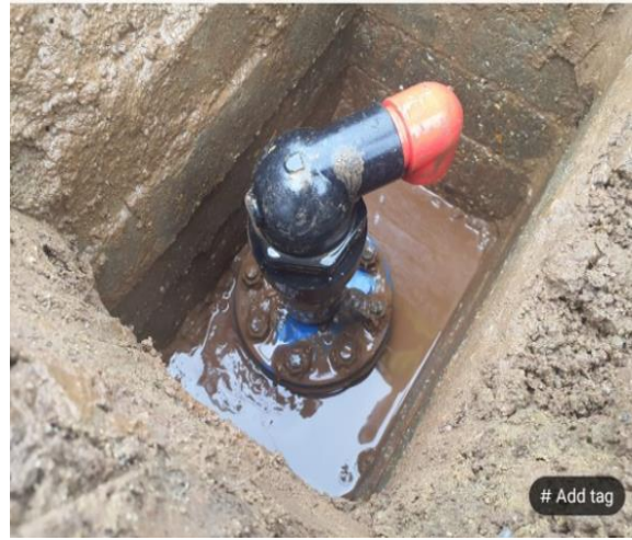
Figure 4 – Chamber dug out
